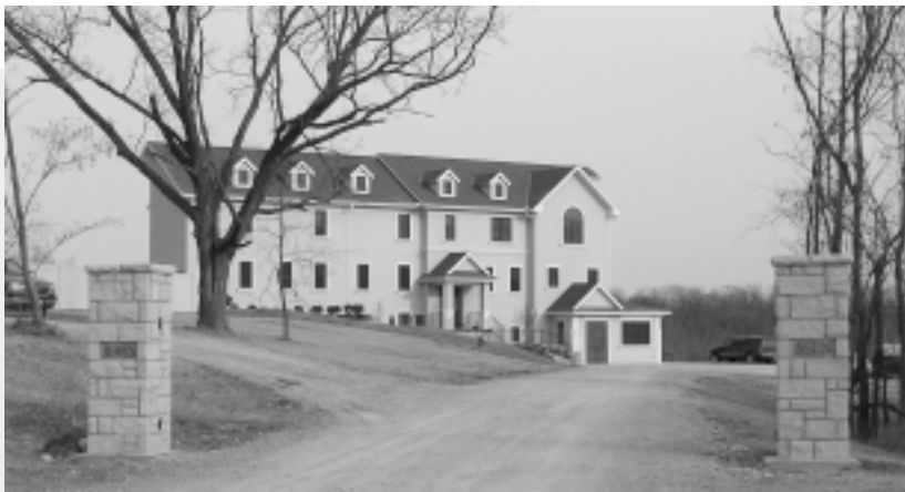
The completed Regina Coeli House, now including stone entrance pillars engraved with the street address on the left and "SSPX" on the right.
