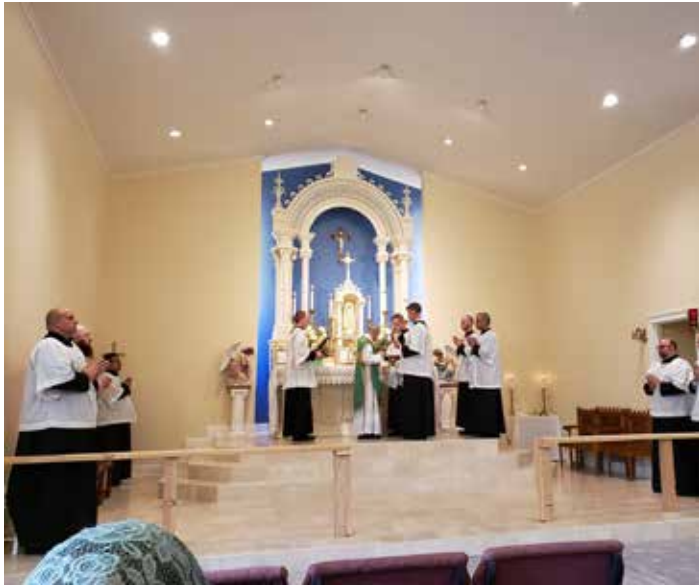
The sanctuary renovations are just about complete at Our Lady of Fatima. The rest of the chapel still needs help, but the sanctuary and the sacristy are finally done!
