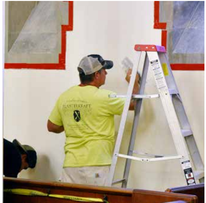
After: The paint was removed from the limestone quoin around the windows. Plaster was floated over the existing walls using “Dryvit” top coat.
